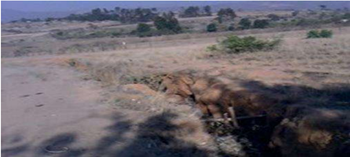
Picture 3.1: Gullies in Ward 11
