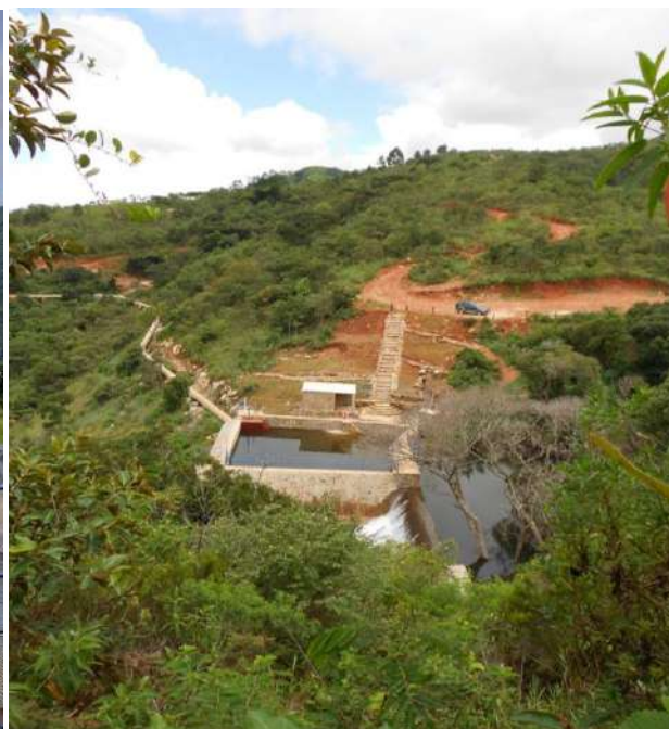
Picture 4.4 Pungwe A hydroelectric power
